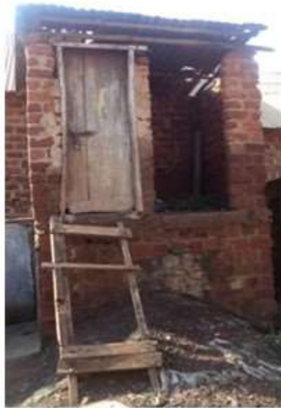
Figure 1: Raised pit latrine with a ladder to ease access
