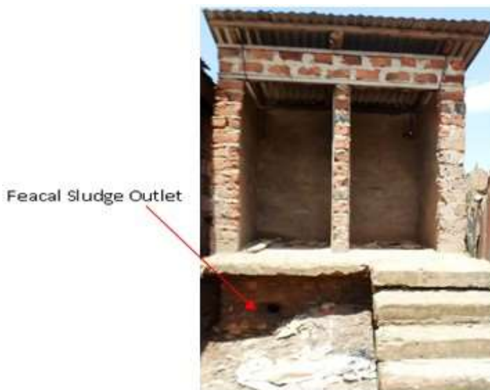
Figure 2: A raised pit latrine with an outlet
